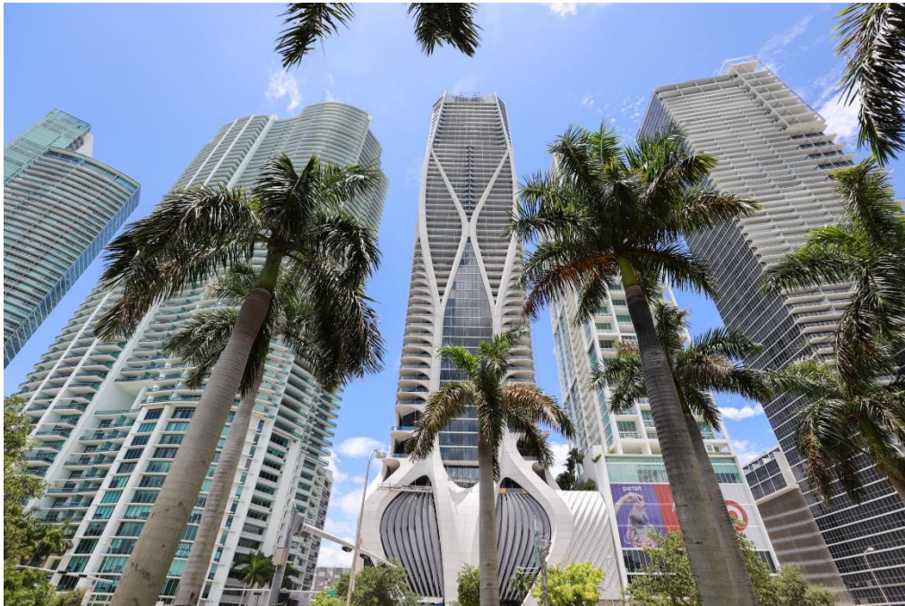
Figure 3.2.a.1: One Thousand Museum building. Project photography copyright Alena Graff 2019
